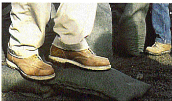
Place each succeeding bag tightly against and partially overlapping the previous one. Compact and shape each bag by walking on it.
